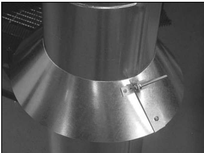
Figure 10.18 Assembling the Storm Collar Around the Pipe
